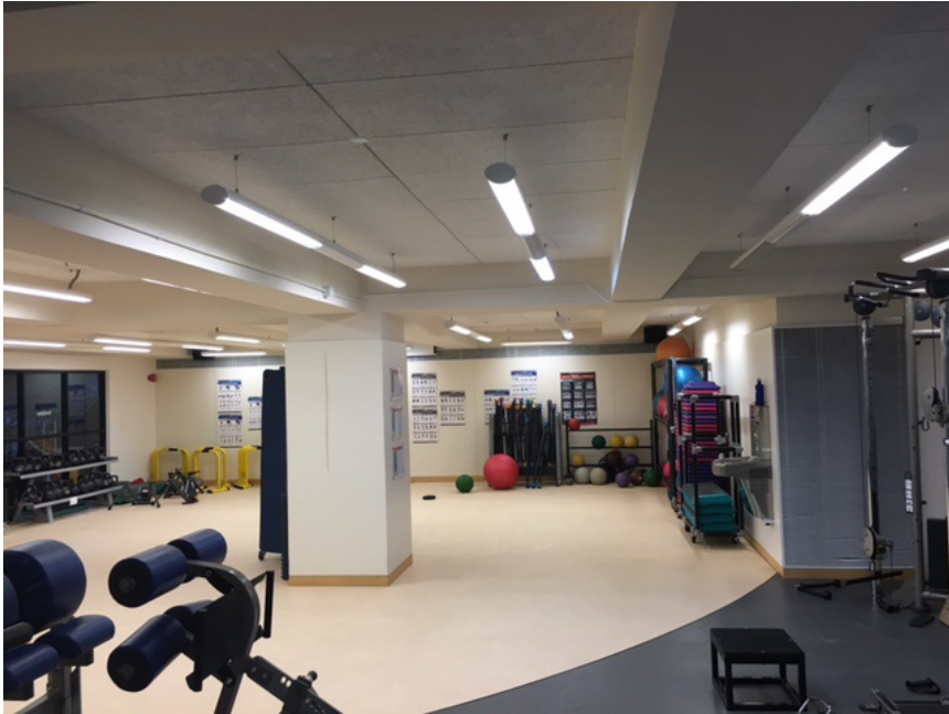
Figure 4. Photo taken from a similar position as Figure 3 providing a view of the new floor area created in the weight room. The center square pillar was the center wall between the squash courts, and the ventilation duct cover on the corner can also be used as a reference point.
