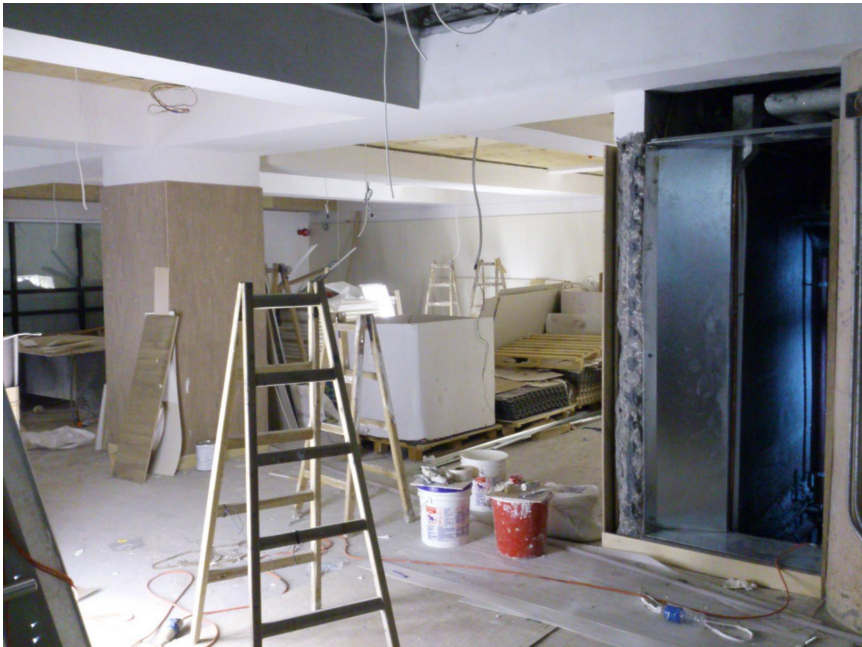
Figure 3. Photo was taken from within the existing weight room. The floor is now complete and the wall that was being removed in Figure 2 is now completely removed. The rough edges of that wall are shown on the right side of the picture, near the air-conditioning duct.
