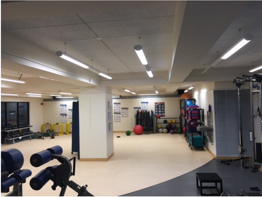
Figure 4. Photo taken from a similar position as Figure 3 providing a view of the new floor area created in the weight room. The center square pillar was the center wall between the squash courts, and the ventilation duct cover on the corner can also be used as a reference point.
